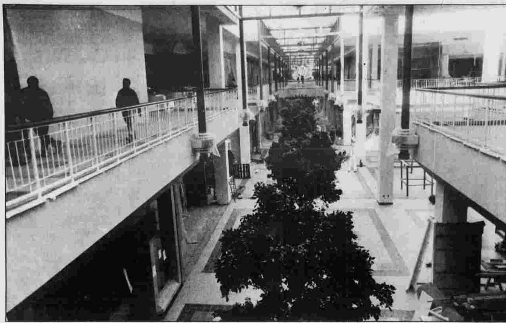
NEAR COMPLETION — The Pavilions at Buckland Hills mall is just about ready for its first shoppers. Sage-Allen will be the first store in the mall to open when it begins business on Wednesday.
